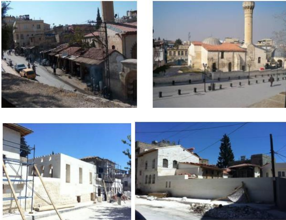
Figure 2.5 Examples of Street Rehabilitation (Source: Teker 2013)
